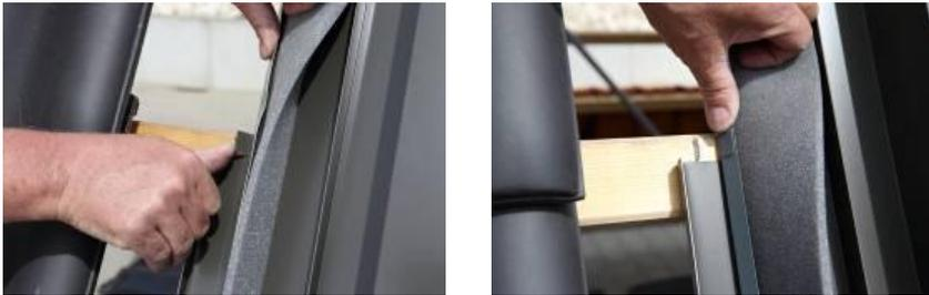
Replace missing tiles and professionally cut to size if necessary. Remove film from self-adhesive roof connection strip and mould strip to shape of tiles.
