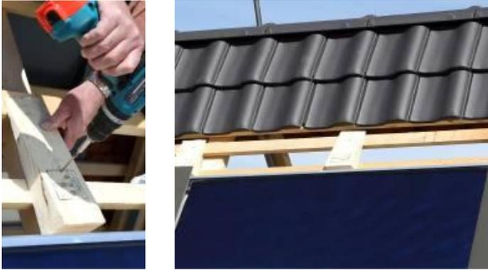
Fit, lock into place and align **upper covering sections of mounting frame** on the left, in the middle and on the right.
