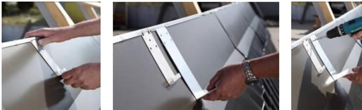
Starting from the left, insert the **flat plate collectors** into the batten brackets and align them so that the gap between the batten bracket and the outer edge of the collector is the same on both sides.
