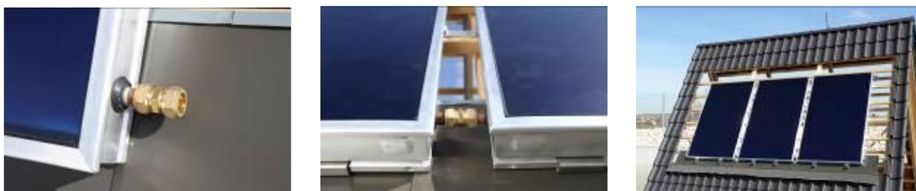
Once all the **flat plate collectors** have been mounted, all the compression fittings (brackets, T-fitting with thermowell, end caps) are to be fitted and aligned. After that, uniformly tighten all the **compression fittings**.
