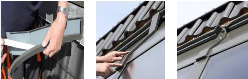
Fix **side sections and upper covering sections of mounting frame** to the battening with sheet fixing hooks, screw on **side sections and upper covering sections of mounting frame** (sheet metal screw 3.5 x 16 mm).
