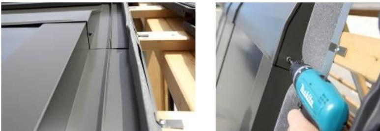
Screw together **bottom sections, side sections and connection strips of mounting frame** (sheet metal screw 3.5 x 16 mm).
