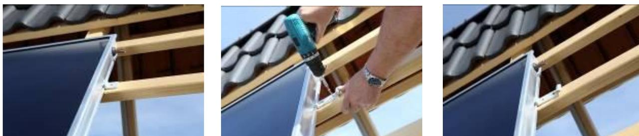
Plug the **compression fittings** into the collector pipes, mount the other **flat plate collectors** as described above.
