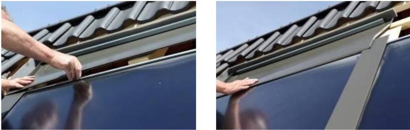
Put sealing tape on the **mounting frame connection strips, short**, hook them in and screw them on (screw with attached washer 4.5 x 35 mm).
