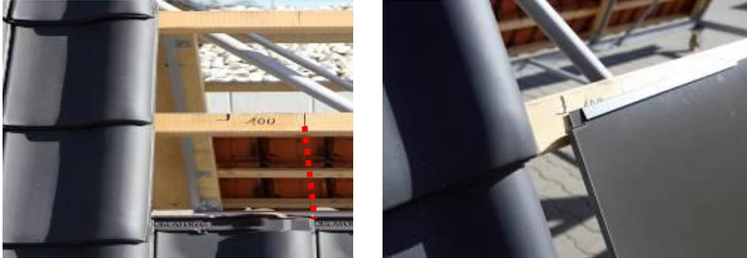
**Metal flashing pieces** are installed from left to right.
