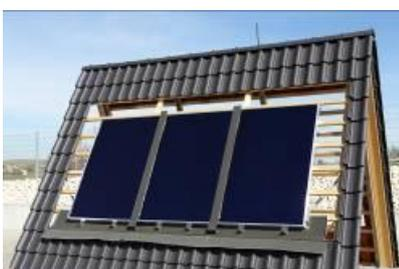
Fit, lock into place and align **bottom sections of mounting frame**.
