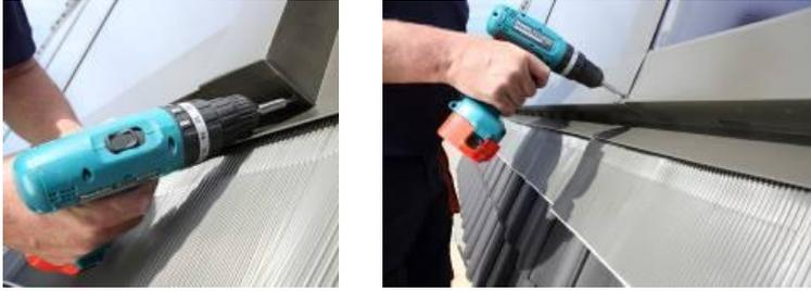
**Bottom sections and side sections of mounting frame** are to be connected to each other on the left and right by flipping over the metal plate.
