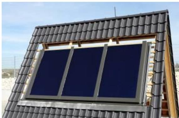
Position and mount **snow load wedges** (chipboard screws 5 x 100 mm). If necessary, mount additional auxiliary lath.
