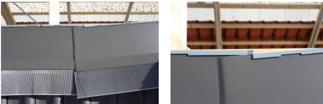
Slide the **batten brackets** and **snow load brackets** into the cut-outs and screw them on (chipboard screws 5 x 35 mm). For an optimum alignment of the batten brackets we recommend fixing a taut string line between the first and the last batten bracket as a guideline.
