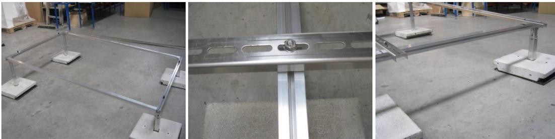
For the installation of the manifold case, mount the clamp in the 1st and 5<sup>th</sup> punching at the upper part of both bars by using one hex socket head screw M8 x 25, one lock washer M8, one clamp and one cage nut each. Screw the clamp loose. Put the manifold case on top and arrange it centrally. The side bars should be positioned between the second and third tube. Then tighten the clamps.
