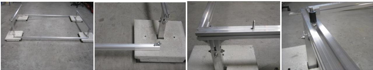
Mount the module side bars (U-profile) and fix them loose with washer and nuts (Fastening set ST-ADM-2BM).
