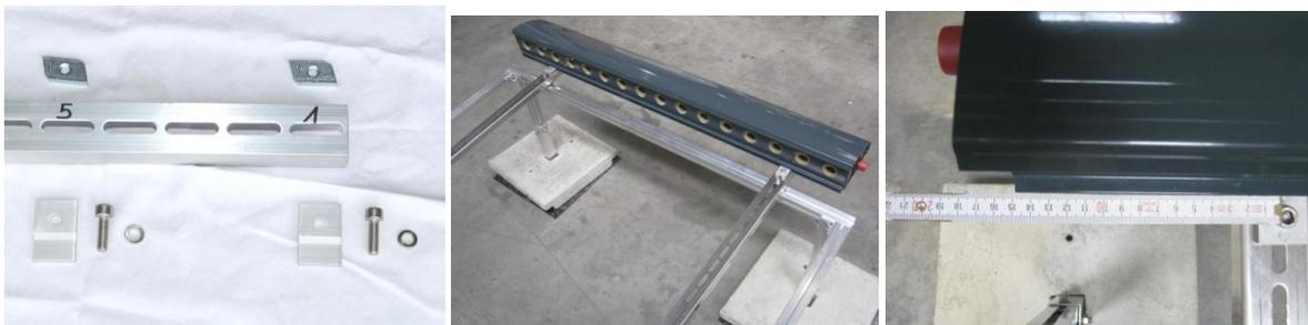
For the installation of the toe bar, mount the clamp in the 1st and 3d punching at the lower part of both bars by using one hex socket head screw M8 x 25, one lock washer M8, one clamp and one cage nut each. Screw the clamp loose. Put the toe bar on top and install the tubes on the left and on the right. Then arrange the manifold case and toe bar parallel to each other. Tighten the clamps.
